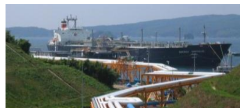
LPG bulk tanker offloading
